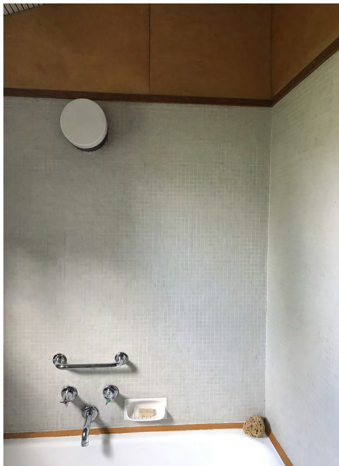
Bathroom: Birch faced ply and mosaic wall finish
